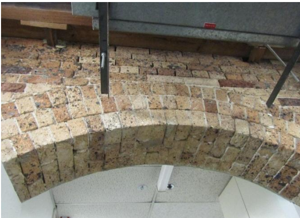
THE CENTRAL ARCH BETWEEN THE STORES HAS MISSING MORTAR AND JOINTS AND REQUIRES SOME ASSESSMENT
