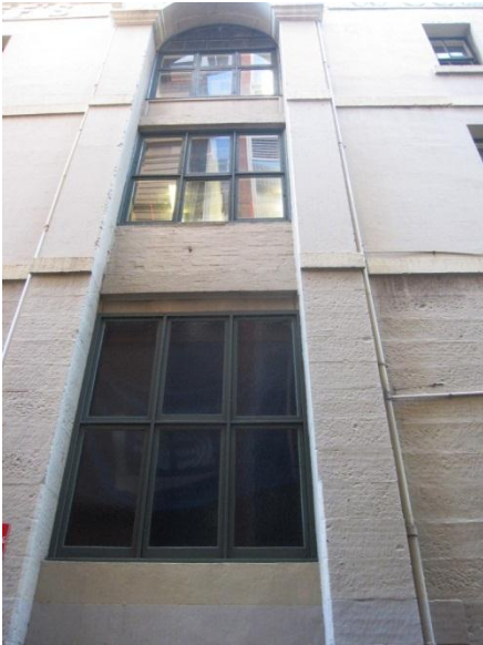
THE MODIFIED CENTRAL LOADING BAY
