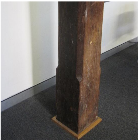
DETAIL OF THE STOP CHAMFERED BASE TO ONE OF THE HARDWOOD POSTS
