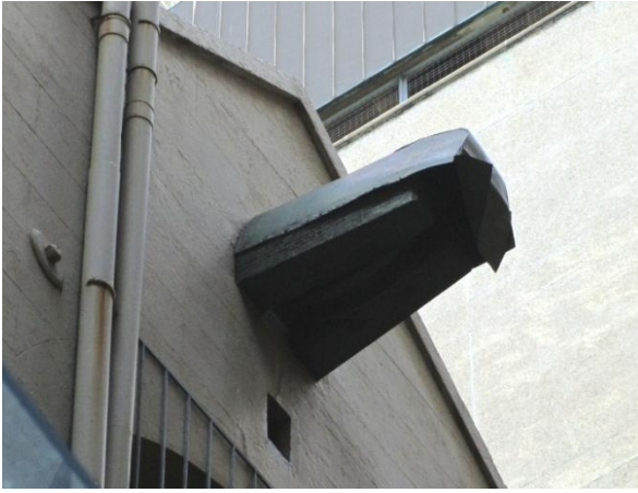
THE NORTHERN BAY CATHEAD PULLEY RETAINS THE STEEL CASING
