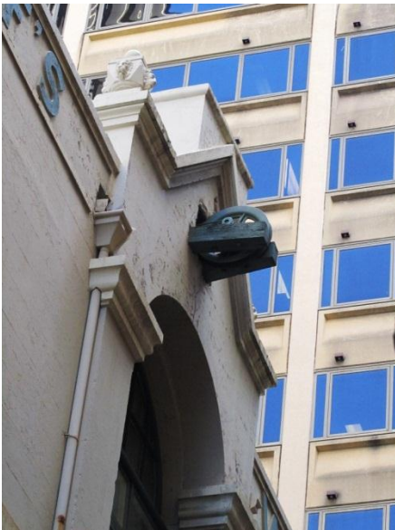
THE GABLED PEDIMENT WITH INTACT CATHEAD PULLEY AND DECORATIVE LION HEAD AND BALL FINIALS – REFER ALSO DETAIL AT RIGHT
