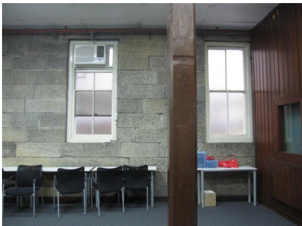
VIEW OF THE INTERNAL SANDSTONE WALL AND ONE OF THE TIMBER POSTS (HAND TOOL MARKS ARE EVIDENT ON THE POSTS).
