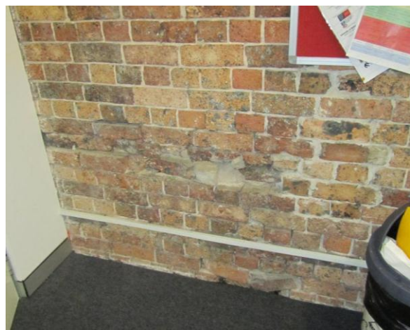
DETAIL OF FAILED AND DAMAGED BRICKWORK AT THE WESTERN END OF THE CENTRAL WALL (NORTH STORE)
