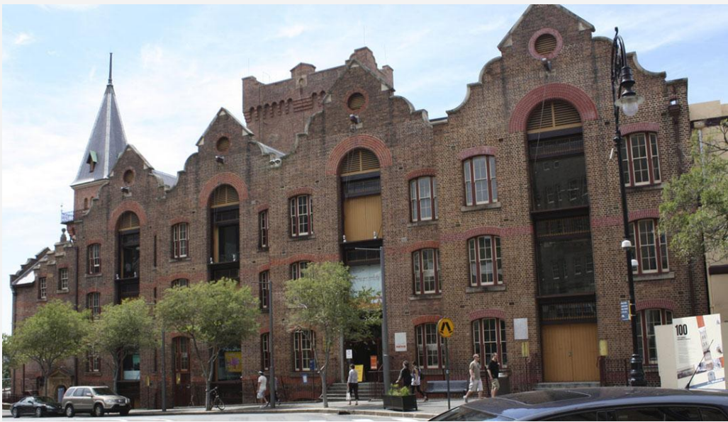
ASN Co Building from George St 2009
