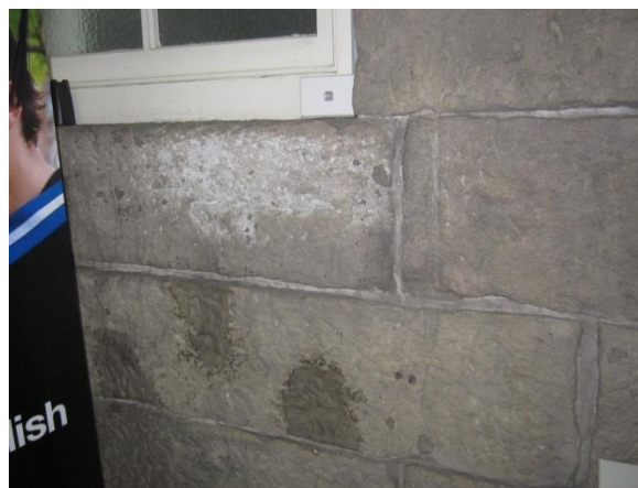
DETAIL OF THE NORTHERN WALL SANDSTONE SHOWING EVIDENCE OF SALT ACTIVITY AND CEMENT PATCHING
