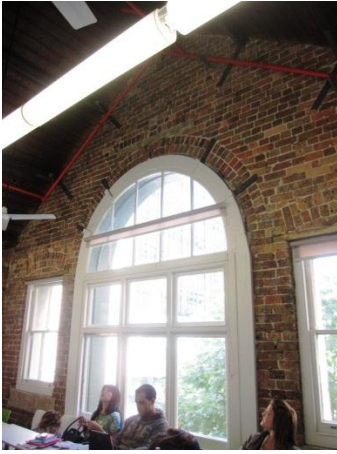
THE EASTERN ELEVATION GABLE SHOWING STEEL REINFORCEMENT OF ARCHED BRICKWORK AND ROOF.
