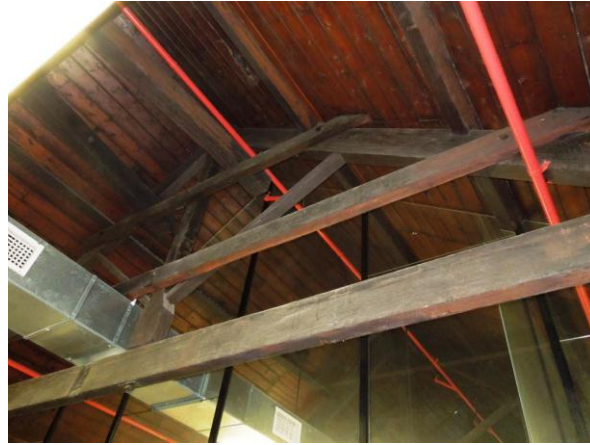
THE KING POST TRUSS ROOF, REINFORCED IN ASSOCIATION WITH THE EXTANT FAÇADE PULLEYS
