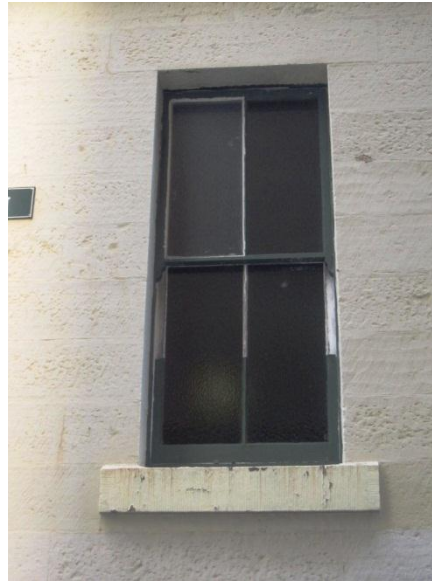
TYPICAL DOUBLE HUNG TIMBER WINDOWS TO THE NORTHERN FAÇADE
