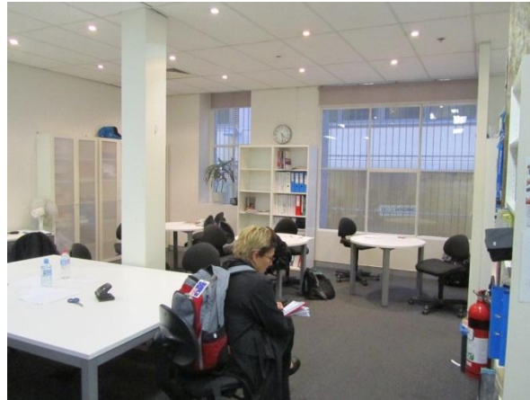
THE REAR TEACHERS/ STAFF ROOM, SHOWING THE STEEL CASEMENT WINDOWS (TO LOFTUS LANE) AND ENCASED HARDWOOD COLUMN (AT LEFT)
