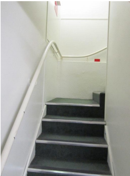
BASEMEN STAIR TO THE GROUND FLOOR
