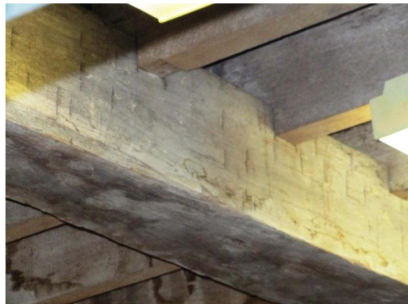
DETAIL OF ONE OF THE SUPPORT BEAMS WITH FLOOR JOISTS OVER. THE BEAM IS HAND ADZED WITH TOOL MARKS EVIDENT (SOUTHERN STORE).
