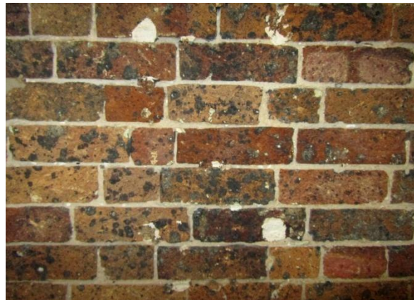
DETAIL OF THE SANDSTOCK BRICK WHICH HAS BEEN DAMAGED IN CONJUNCTION WITH THE REMOVAL OF RENDER AND FINISHES
